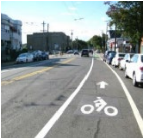
On-Road/Signed Bike Route
